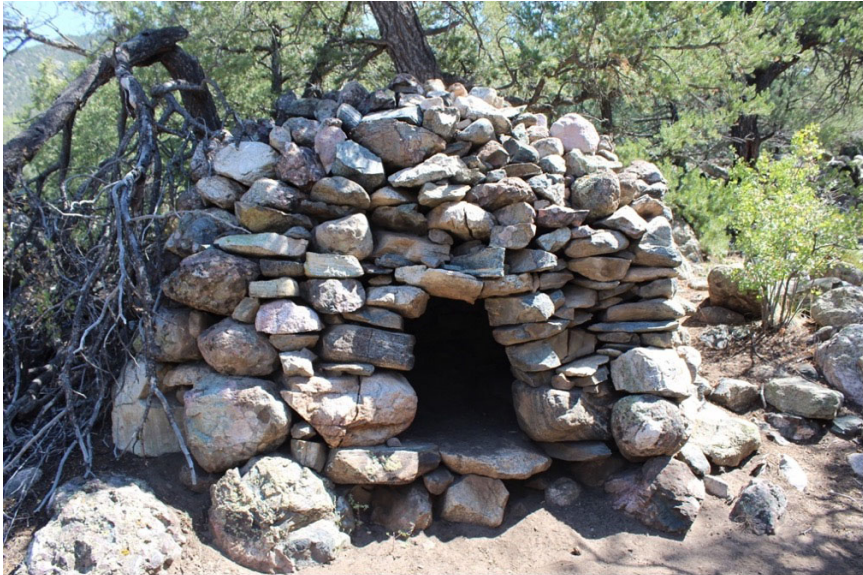
Figure 4. Crestone Structure #4 (Piñon House).
