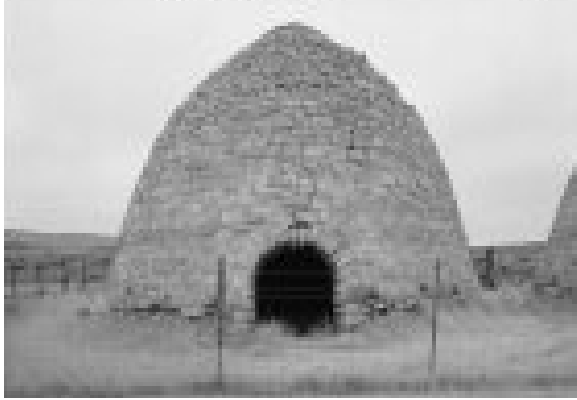
Figure 8. Piedmont charcoal kilns in Uinta County, Wyoming, constructed in 1869. (Photograph courtesy of the Historic American Buildings Survey, Library of Congress, call number: HABS WYO,21-PIED,1-)
